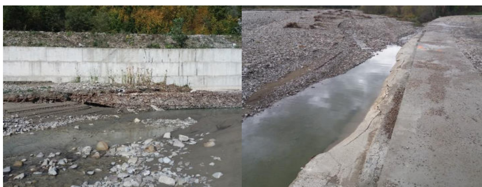
Figure 29. Degradation by lowering the level of the trough of the works of gabions covered with concrete with concrete (author's photo)
