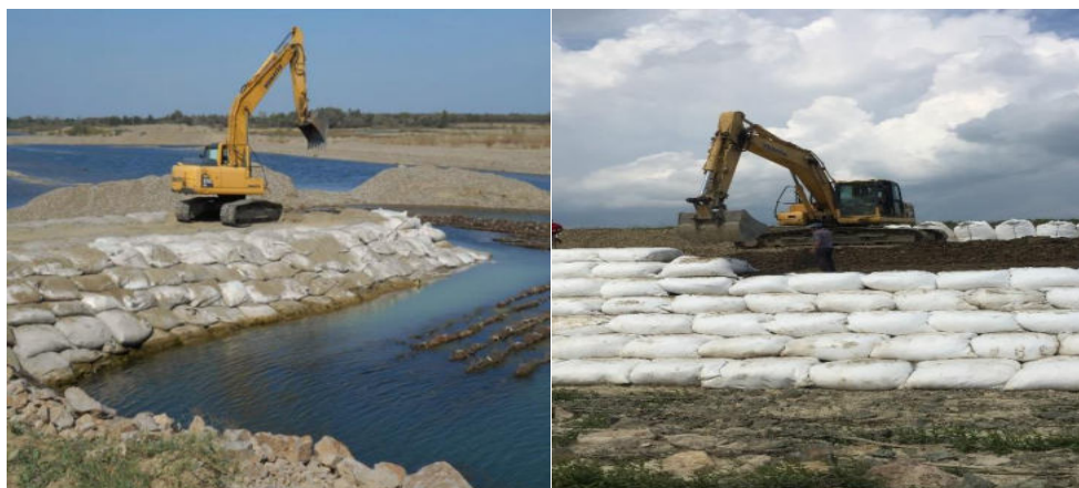
Figure 18. Placement of geocontainers (author's photo)
