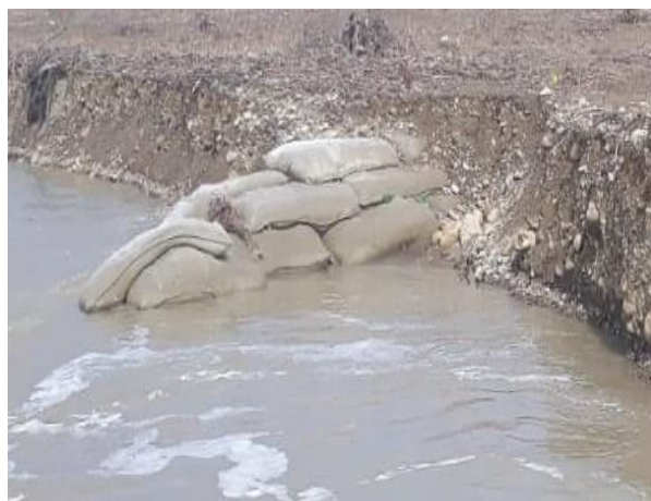
Figure 36. Degradation by flattening and bending
