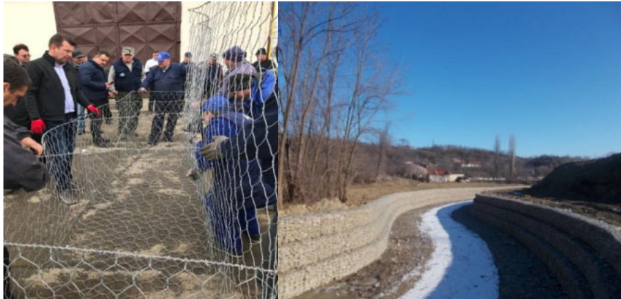
Figure 8. Assembling of alternative gabions (author's photo)
