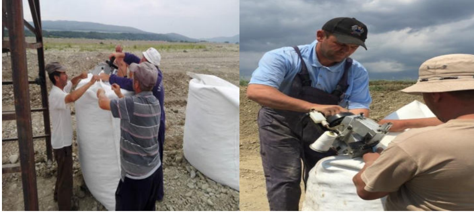
Figure 16. Geocontainer sewing operation (author's photo)
