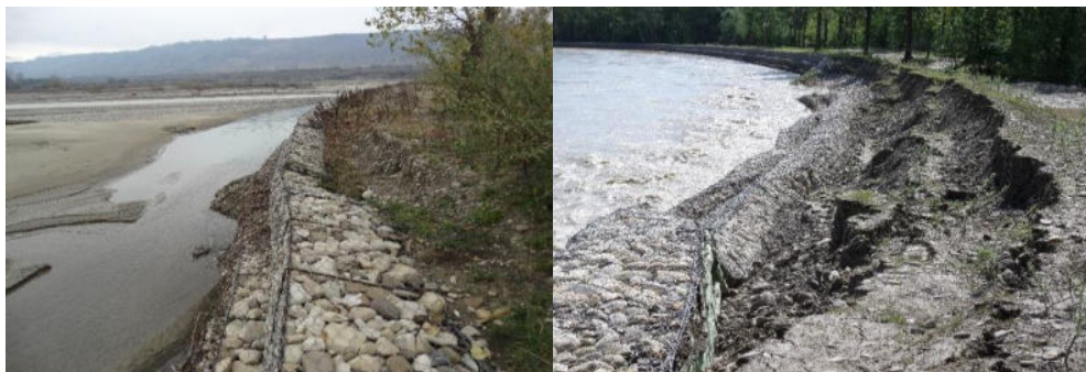
Figure 27. Gabion work degraded by sliding (author's photo)
