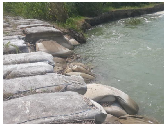
Figure 41. Degradation of the geocontainer work by moving the geocontainer - transversal work (author's photo)
