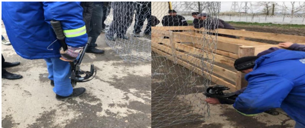
Figure 6. Attaching the staples using pliers manually (author's photo)
