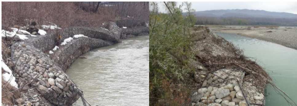
Figure 26. Overturned gabion work (author's photo)
