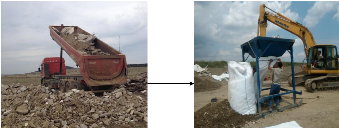
Figure 100. Use of debris to fill geocontainers
