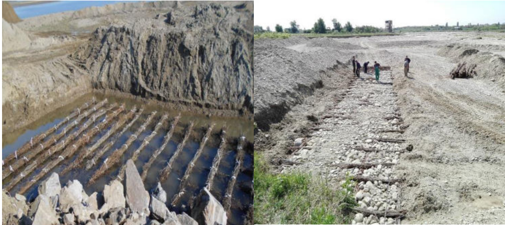
Figure 14. Site preparation, fascine mattress ballasted with rock (author's photo)
