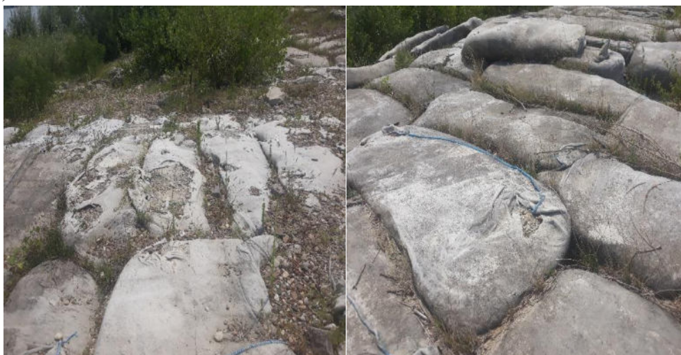
Figure 47. Degradation caused by float transport (author's photo)
