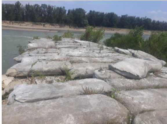
Figure 43. Degradation by exceeding the level of the work (author's photo)
