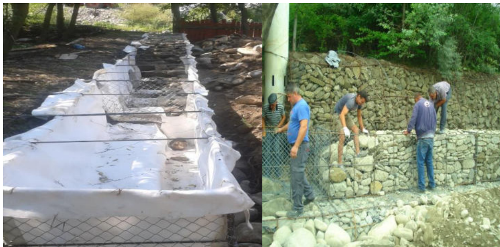
Figure 13. Filling the gabions with rough stone (author's photo)
