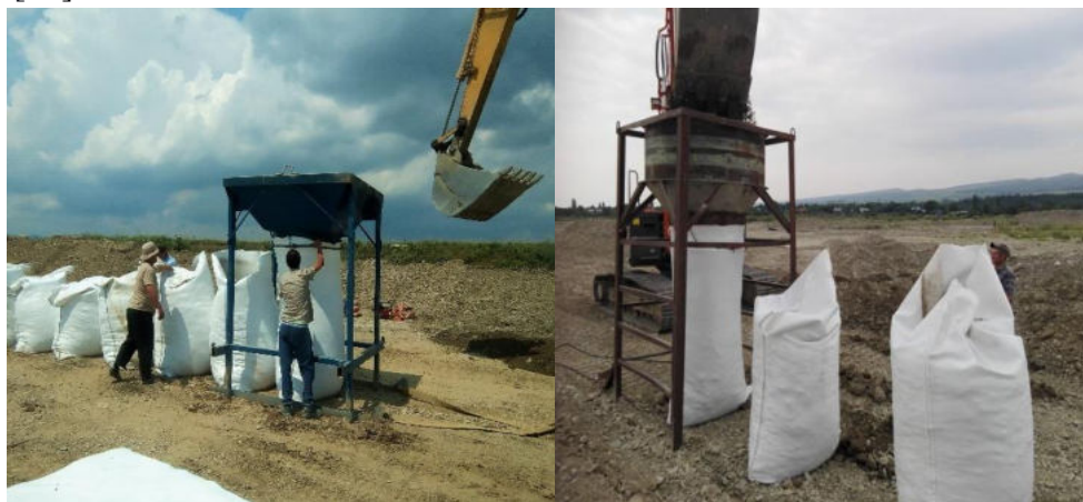
Figure 15. Bag filling operation (author's photo)
