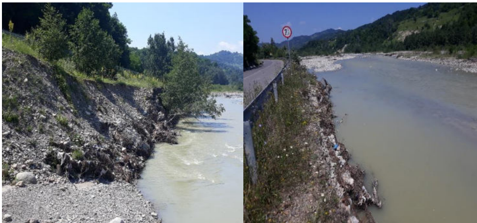
Figure 31. Degradation caused by the transport of alluvium and floats (author's photo)
