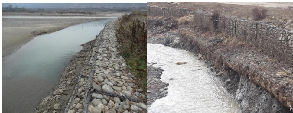
Figure 28. Degradation by lowering the level of the trough of simple gabion works (author's photo)
