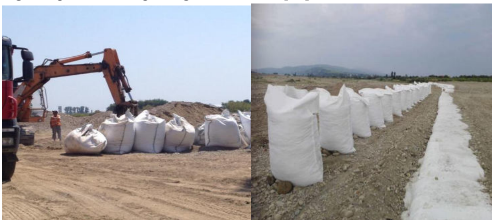
Figure 17. Preparation of geocontainers for placement (author's photo)
