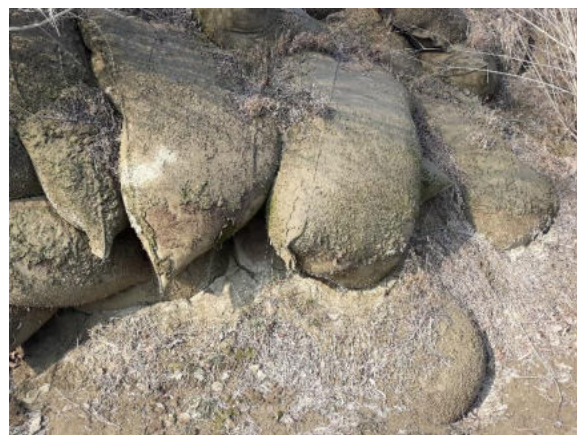
Figure 39. Degradation of the geocontainer work by decreasing the elevation of the basin - situation on site (author's photo)
