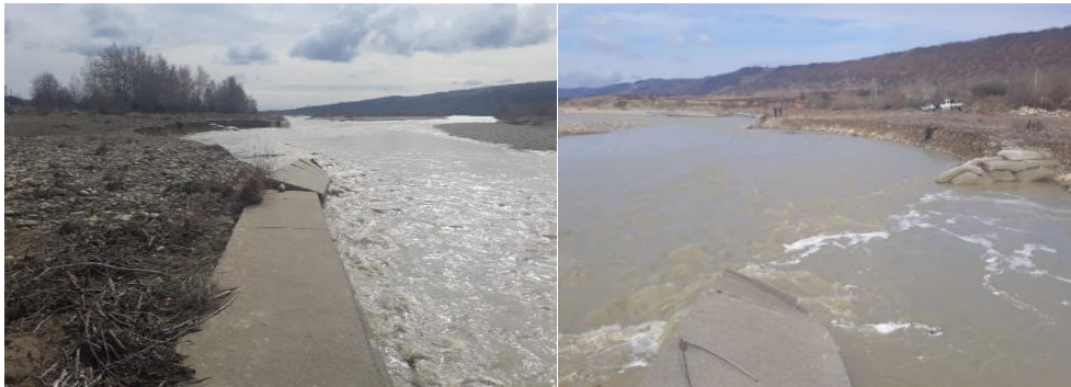
Figure 25. Gabion work covered with overturned concrete (author's photo)
